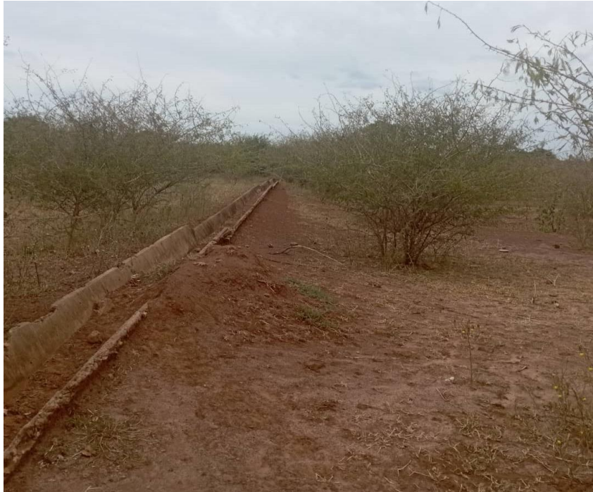
Figure 40: Deserted Sengwa Irrigation Scheme in Gokwe South
